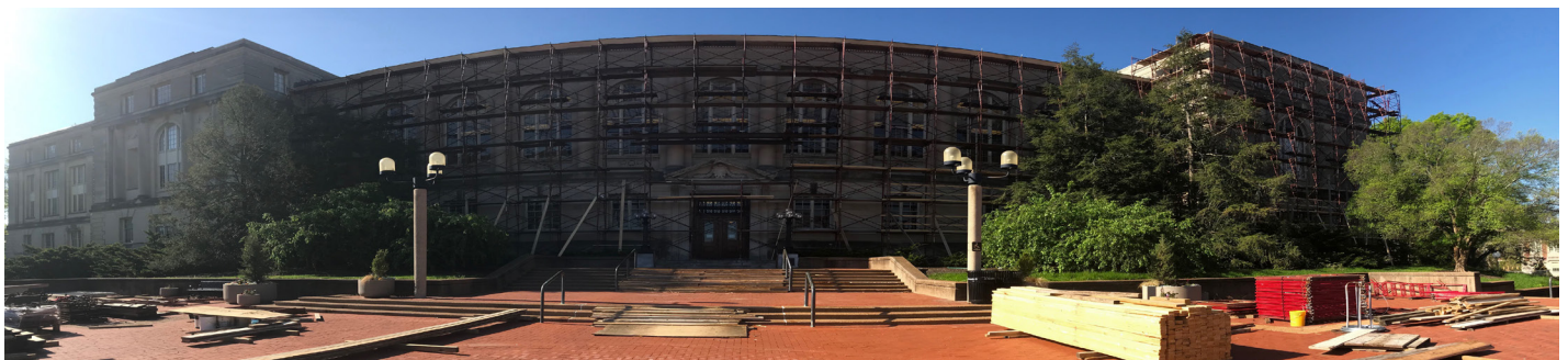
Many of the historical windows in Ellis Library are being replaced or renovated this spring. The project, which is expected to cost over $2 million, impacts the original 1914 building and the 1935 addition. Photo by Kate Anderson.
